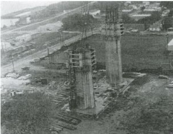
6.1.4 Pier four was the first pier to be finished, mainly due to its ease of access. For the footing a sheet pile cofferdam was installed and then 160 were driven in to the ground. Once this had been done the footing was then completed in one big pour. Then it was a simple case of building the pier shafts and the strut.
