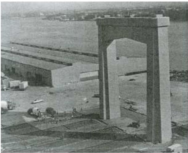
6.1.2 The second pier is the most complicated of all the piers and as a result would have been started first as it would take a long time to construct.
