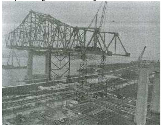
The cantilevers were then simply continued out with the help of scissor jacks. This meant that during construction the cantilevers were actually longer than when the bridge is finished. Then to close the structure a process called "swinging the span" allowed the scissor jacks to be relaxed and removed which changed the bridge from two long cantilevers to being two shorter cantilever arms supporting a central span.
