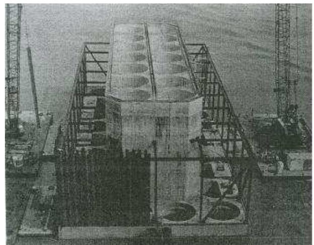
To protect both ships and the bridge pier a timber fender was constructed around the pier. Using pinewood coated with creosote coal-tar did this.
