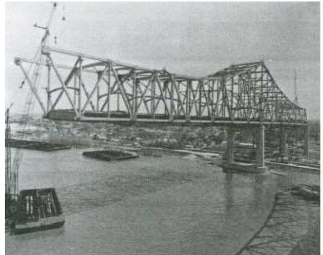
The New Orleans anchor span was next to be started, this used a balanced cantilever method. Whilst the shorter span was being constructed the longer span was also erected at the same time. After an adequate stage of construction had been reached, the contractors went back to Pier three to erect the steel towards pier two, cantilevering the span out into the river. Steels were lifted into place using the lift on the barge.
