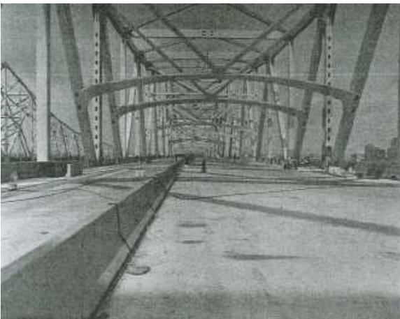
To reduce the dead load of the bridge steel barriers were designed and erected to divide the 4 standard vehicular lanes up with the two HOV lanes. So the next process was
