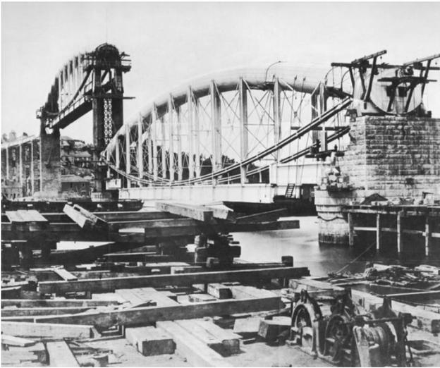
**Figure 17:** Photo of the 2 span being lifted into position
