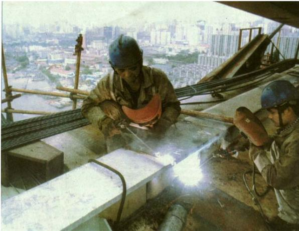
**Figure 11:** Welding of the steel arch. Ref [9]
