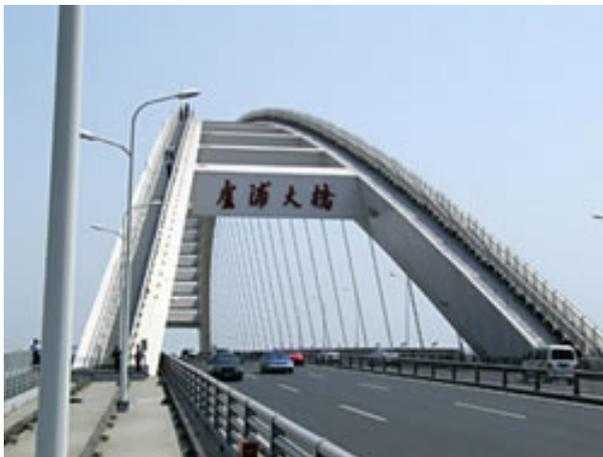
Figure 3: Arches protruding out of the deck. Ref. [3]
