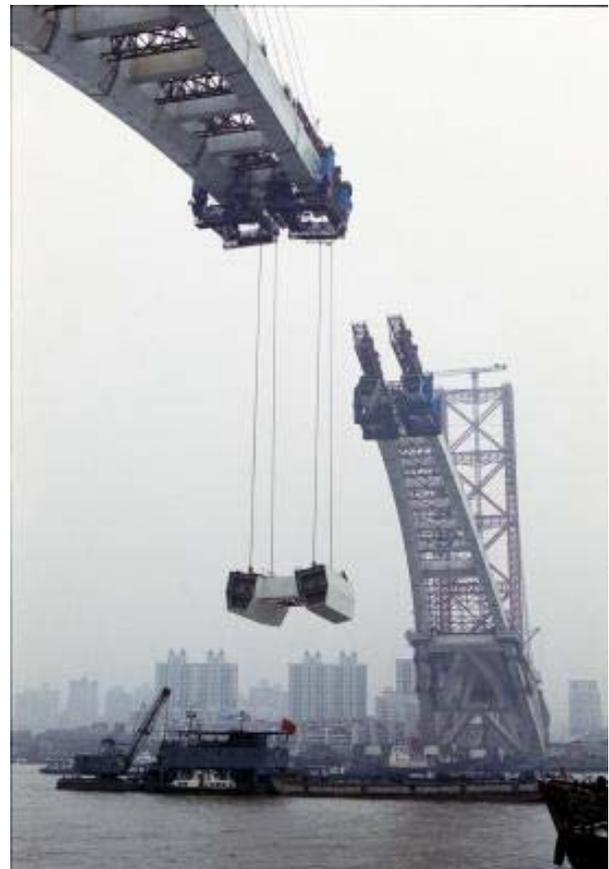
**Figure 10:** Lifting the arch sections into position
