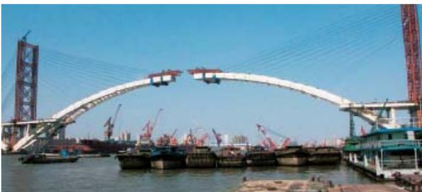
**Figure 9:** Cable-Stayed Cantilever Construction.
