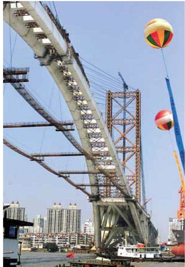
**Figure 12:** Horizontal cable installation. Ref [9]
