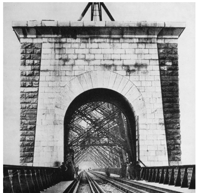
Figure 6: Looking through the cantilever abutment showing the ordered brickwork and bracing.
