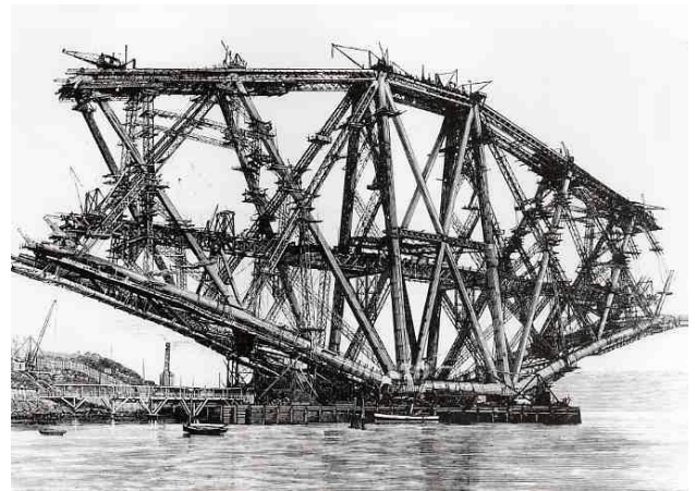
Figure 4: A construction photograph showing how the cantilever arms were built equally on each side.
