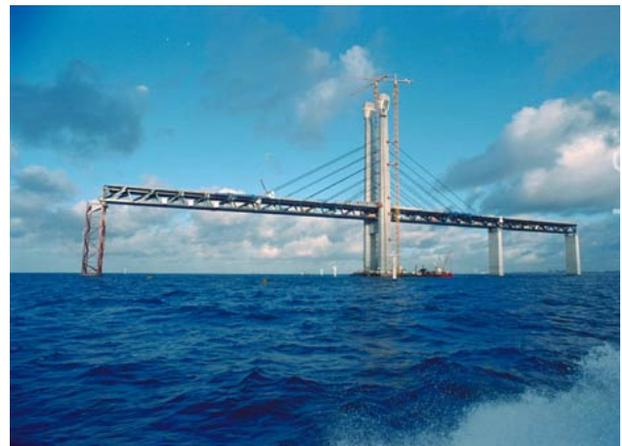
Figure 7: Half of main span with temporary pier
