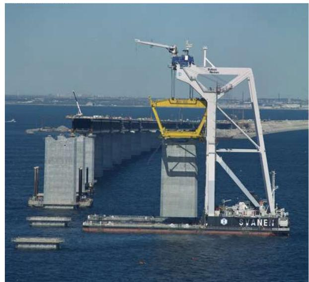
**Figure 5:** 'Svanen' placing a pier in the bridge line
