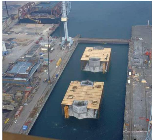
**Figure 4:** Pier caissons ready to be floated to bridge line
