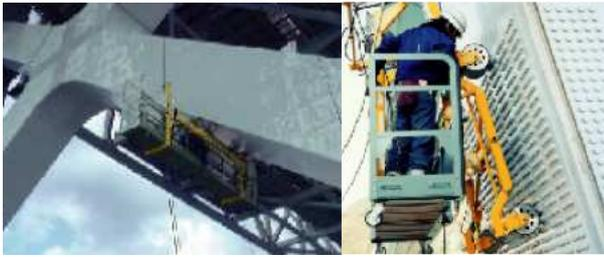
Figure 18: Magnetic wheel gondola work on (a) tower wall and (b) diagonal and horizontal member.
