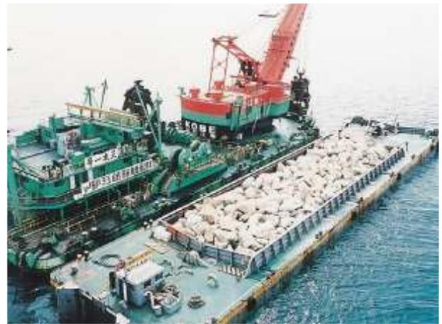
Figure 2: Protecting of the caisson against scouring
