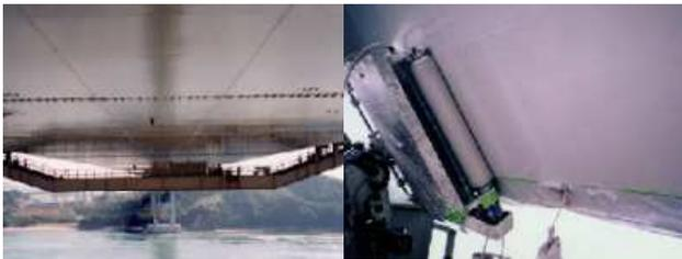
Figure 19: (a) Moveable maintenance platform (b) Painting robot
