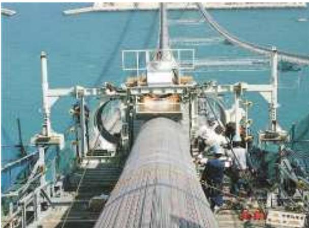
Figure 4: Installation of cable strand
