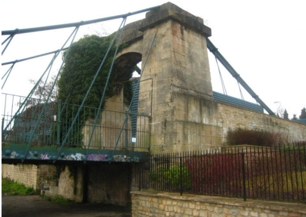
Figure 5: View of the northern pier
