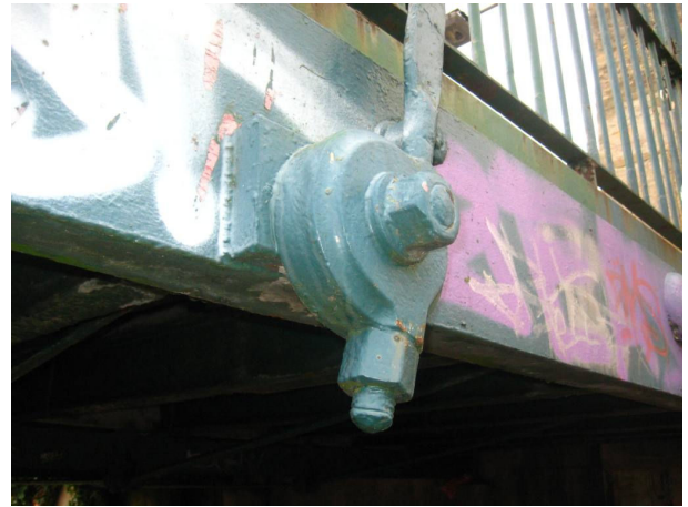
Figure 6: Hanger connection detail
