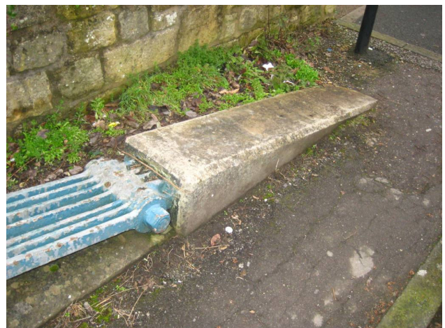
Figure 4: Anchor blocks at the southern end of the chain
