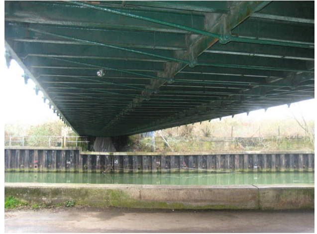
Figure 9: View of underside from towpath
