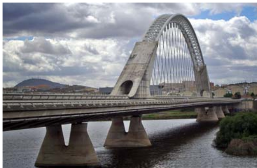
Figure 6: Concrete Abutments of Lusitania Bridge
