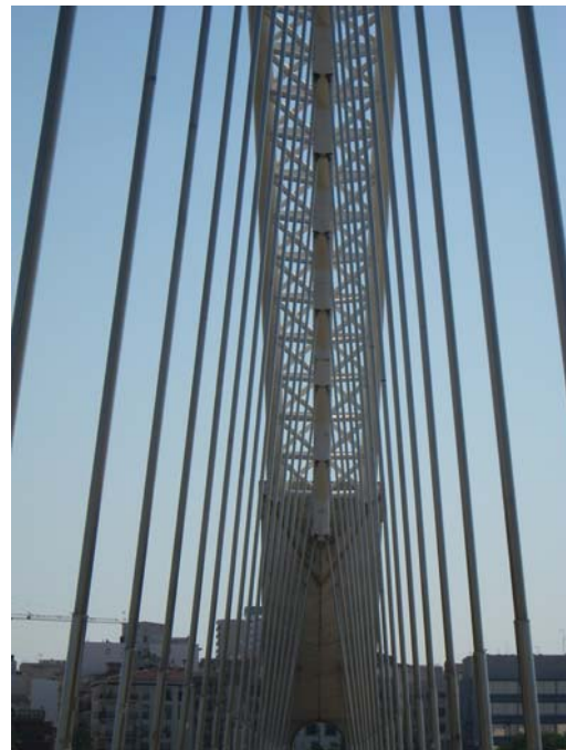
Figure 7: Steel Rods and Arch Structure
