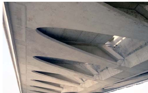
Figure 5: Structural Wings of Deck
