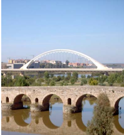
Figure 2: The old Roman La Akazaba Bridge and the new Lusitania Bridge in the background
