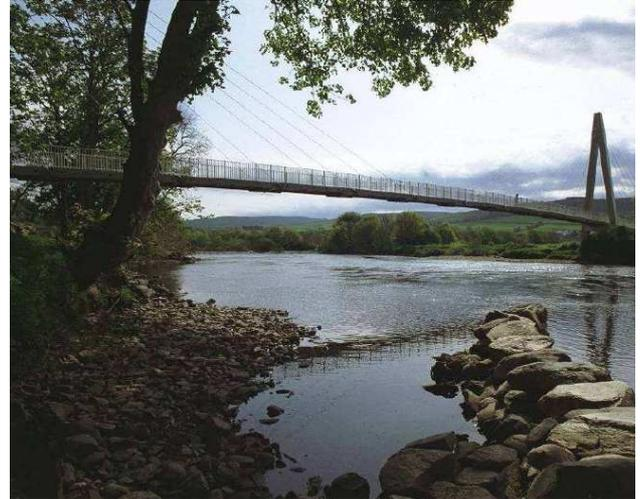
**Figure 3:** Cables designed in a fan arrangement [5]
