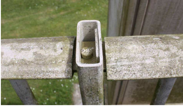
Figure 12: Frictional joint [5]
