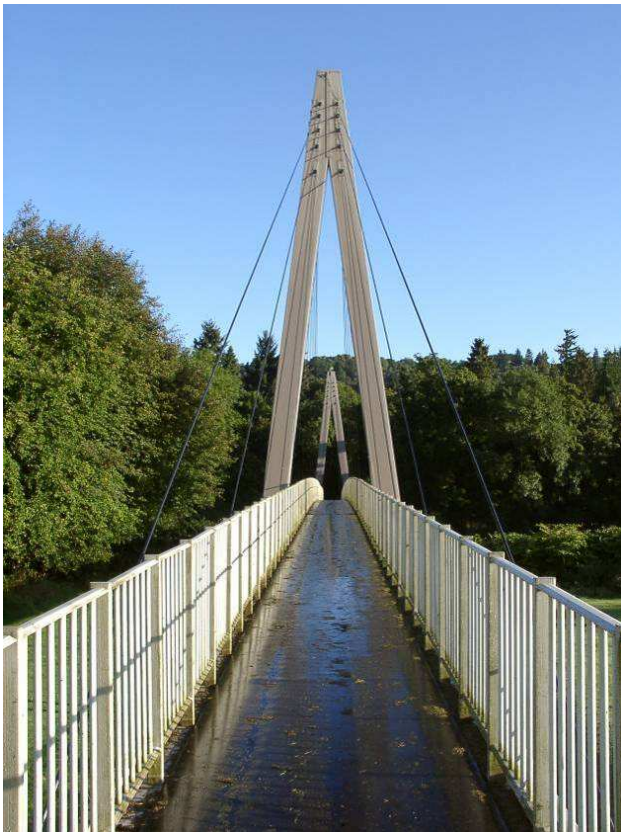
Figure 2: Walking over the bridge [4]
