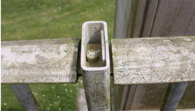
**Figure 12:** Frictional joint [5]
