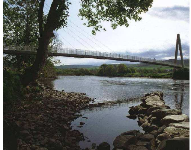
Figure 3: Cables designed in a fan arrangement [5]
