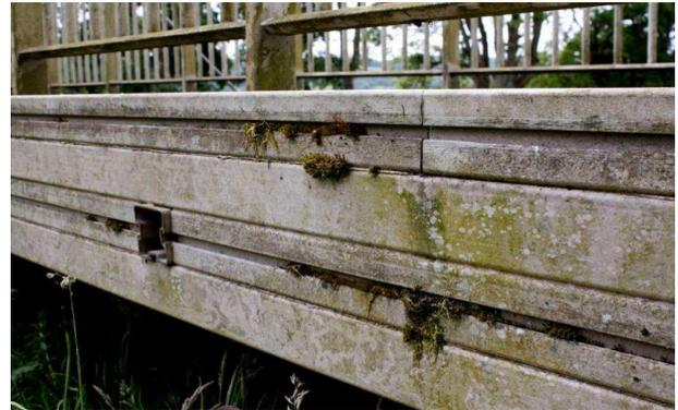
**Figure 13:** Mould and lichen growth [5]
