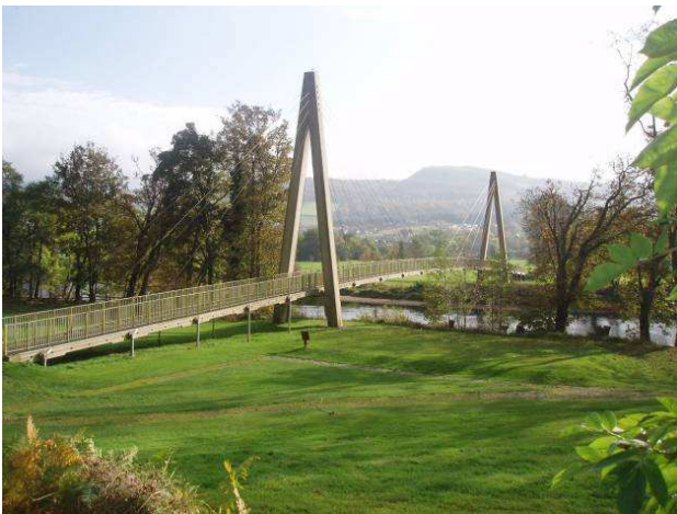
Figure 1: The Aberfeldy footbridge [2]
