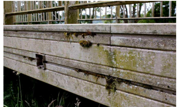
Figure 13: Mould and lichen growth [5]
