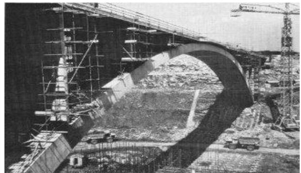
**Figure 15:** Spandrel scaffolding and formwork; [1]
