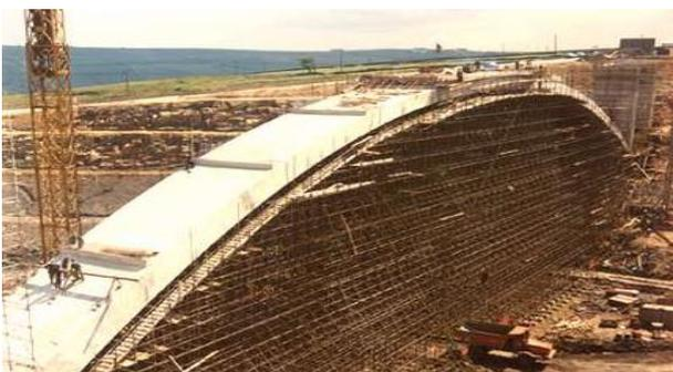
**Figure 14:** Temporary arch centring framework with precast arch sections and spandrel joints; [4]
