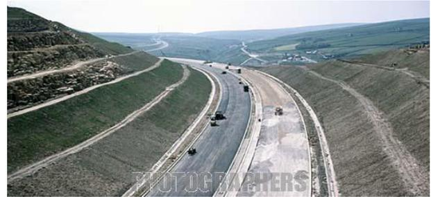
**Figure 12:** Deanhead cutting being profiled in 1970
