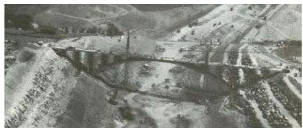
**Figure 16:** Ariel view of bridge taken when the deck was craned into position
