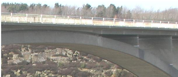
**Figure 2:** Close-up of the deck and spandrel columns
