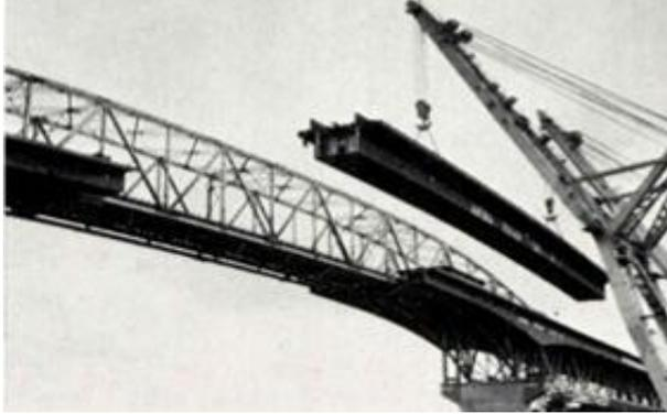
Figure 9: Steel box sections during construction
