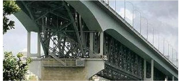
Figure 4: Truss elements at oblique angle
