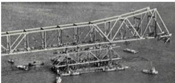
**Figure 18:** Transportation of trusses
