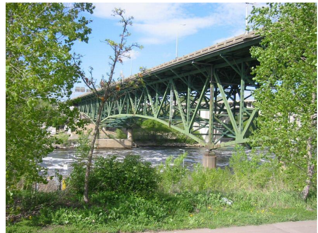
Figure 2: Bridge 9340 before its collapse
