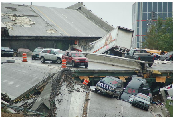
Figure 3: Bridge 9340 immediately after its collapse
