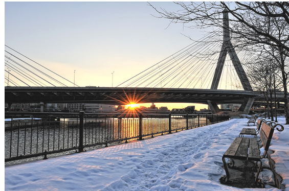
Figure 1: Eastern view of bridge
