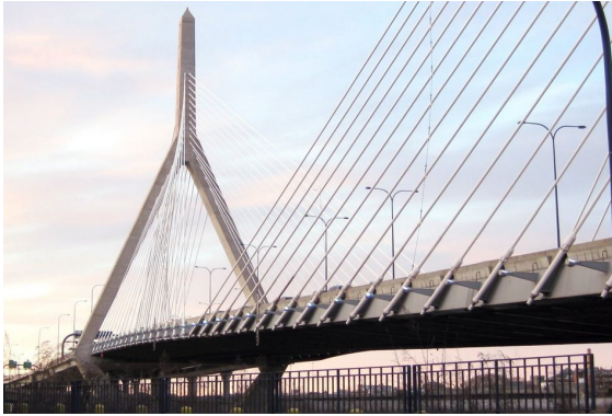
Figure 2: Western view of tower and bridge deck
