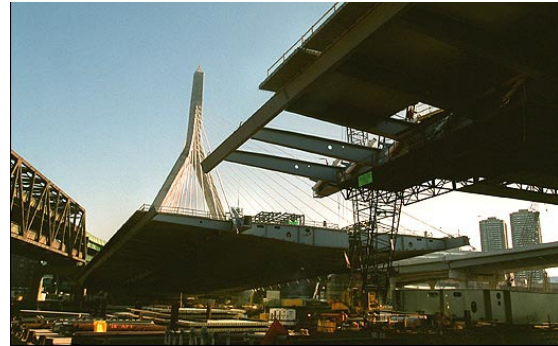
Figure 10: Cantilever construction of main span deck
