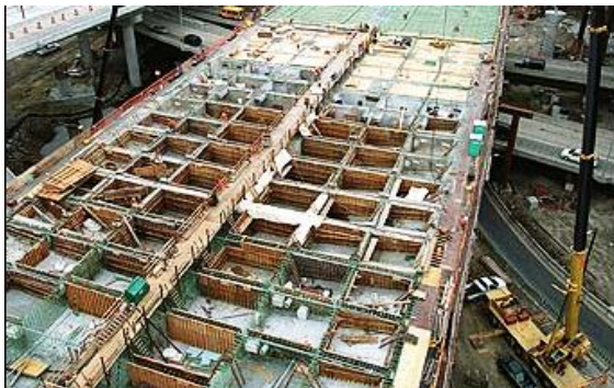
Figure 9: Construction of north back span
