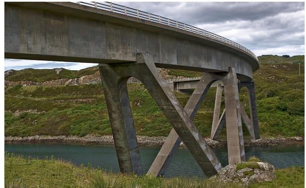
**Figure 3:** Photo showing the supports blending into the gneiss bedrock, the crossing of the supports, the joints from the supports to the deck, the thickness of the deck and the weathering of the concrete
