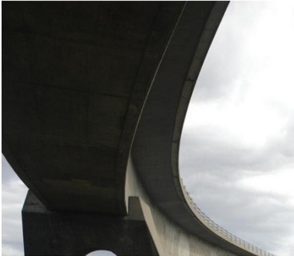
**Figure 6:** Photo of the underside of the bridge deck, showing evidence of incremental launching
