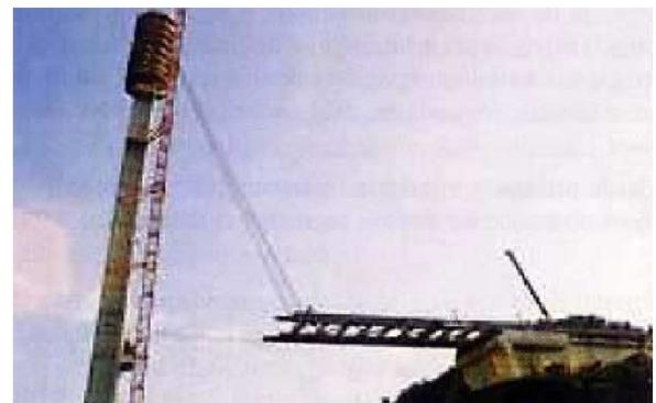
**Figure 16:** Bridge construction, incremental launching [2]
