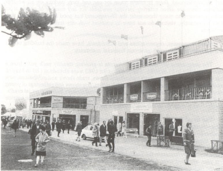
The Unigate Demonstration Theatre and the Cheddar Cheese Restaurant and Exhibition Hall, which form part of over 71,000 sq. ft. of undercover exhibition and conference facilities on the Royal Bath & West Showground.
