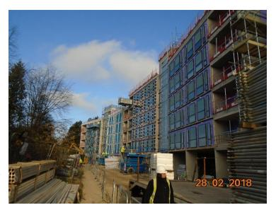
Our stone cladding panels have now been delivered to site, and fitting has now commenced. This along with even more windows now installed means the façade of the building is taking shape, and will soon start to resemble the finished product.
