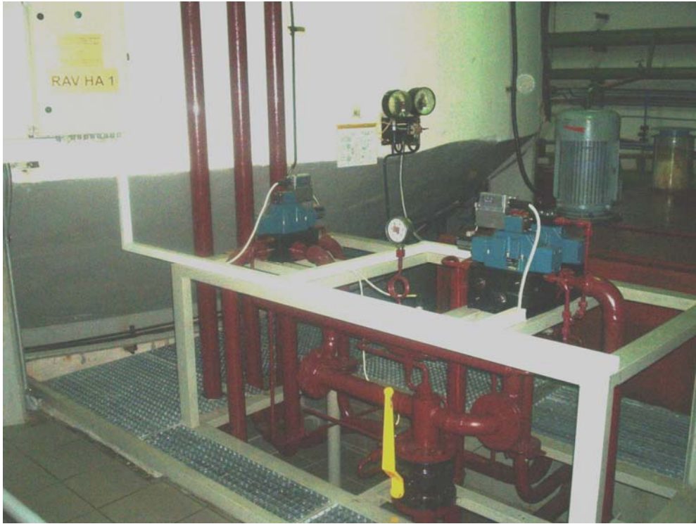
Figure 6 New speed governor hydraulic assembly front view
