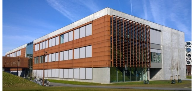
Figure 1: The considered case study university building (Jradi et al. (2017)).
