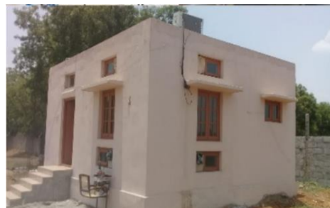
Figure 6: Residential Test Bed
