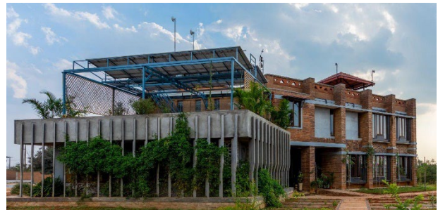
Figure 1: The Experimental Building
