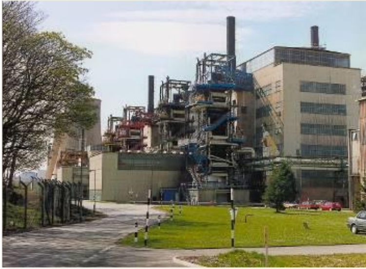
Magnox - Calder Hall
