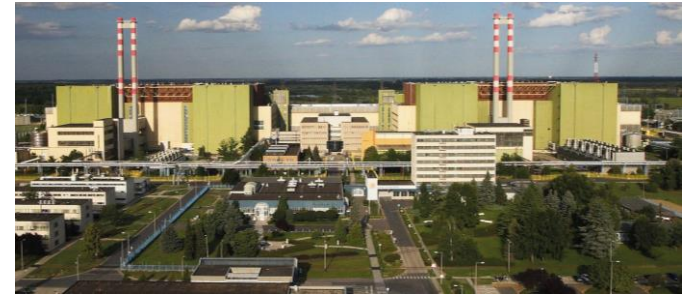
Paks Nuclear Power Station, Central Hungary
