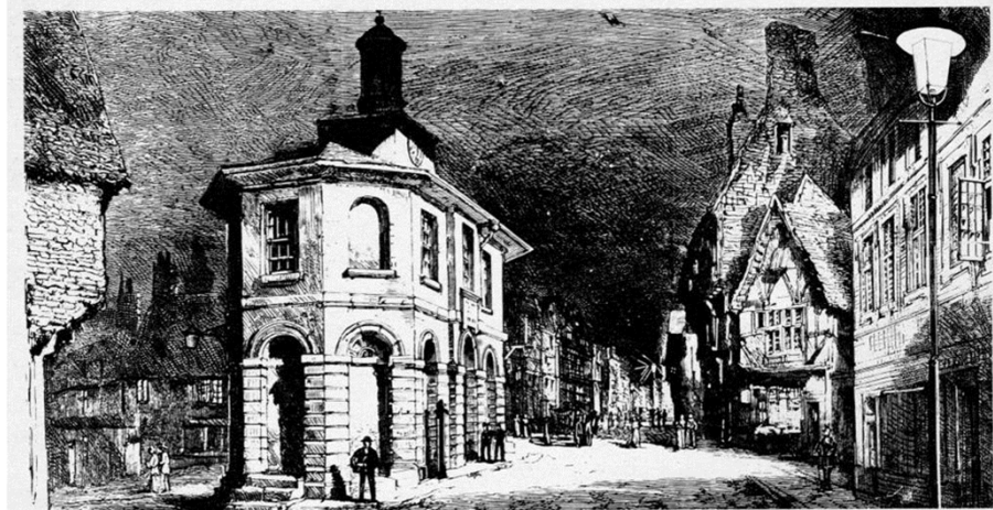
Incandescent lamps shone from three 24 ft high posts. The light that flooded the cobblestones of Godalming signalled the birth of the electricity supply industry.
