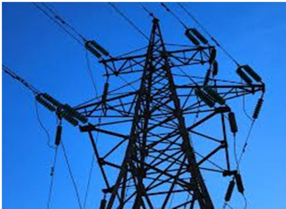
Condition of the supply System
