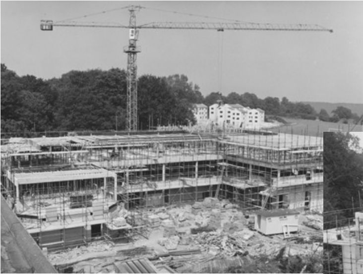
3 East under construction
