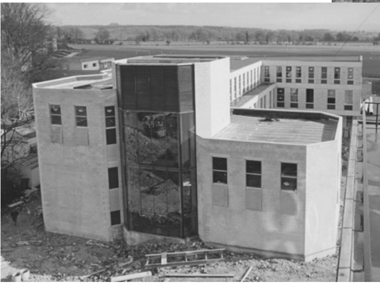
3 East nearly completed
